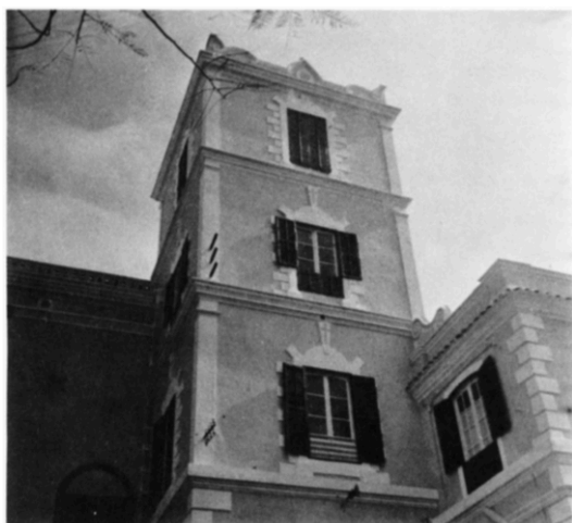
Fig. 6. Belfry, and part of administration block and sanctuary chapel (photo: author 1956).
